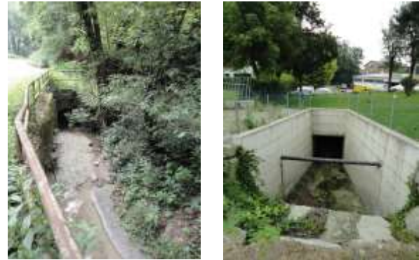
Examples of piped sections in the intervention area
